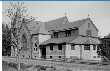
1889 view of church from Maple Ave.
