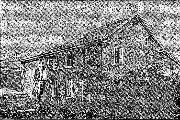
THE MOORE FURMAN HOUSE: DEMOLISHED
