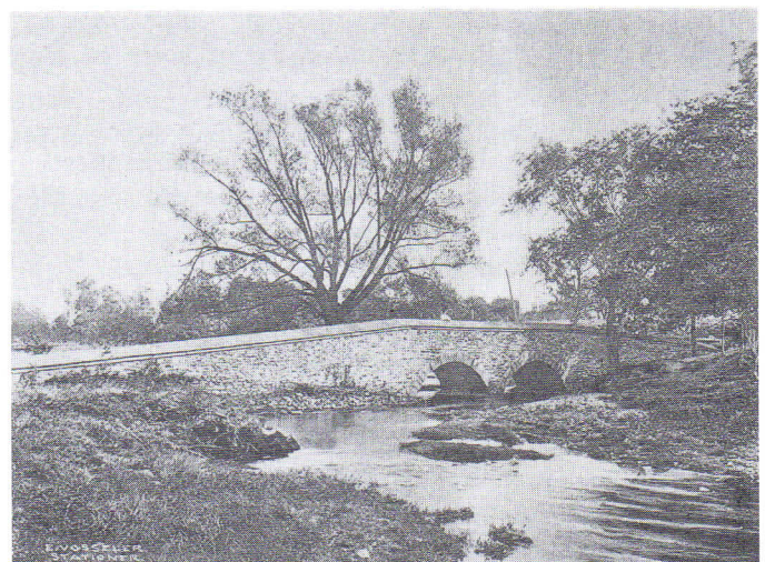
Pictured above is a stone arch bridge near Flemington spanning the Neshanic River, built circa 1834. See above request for assistance in securing information on Hunterdon County stone arch bridges.
