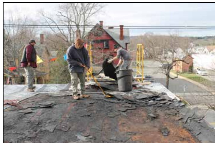
Sam Tippet and crew scraped off five layers of built-up roofing.
