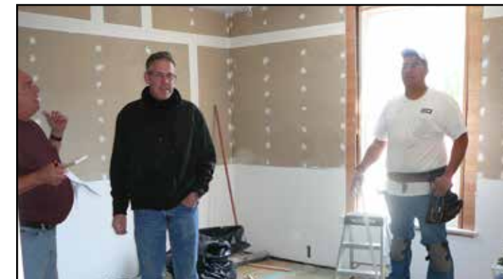
Building the Second Floor Exhibition Space
