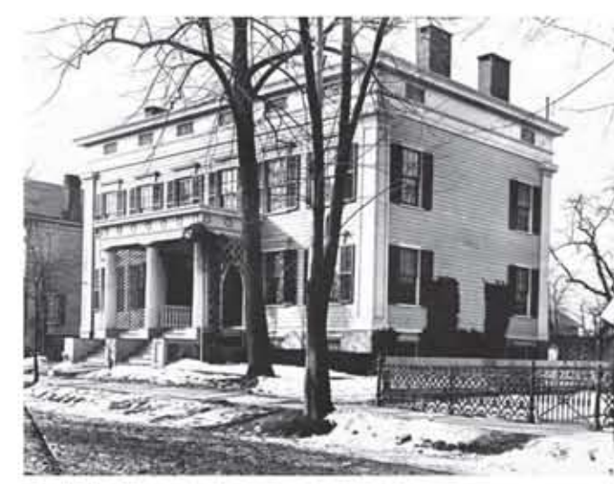
23 Reading/Dorf residence 1845 Designed by Mahlon Fisher for two brothers, this impressive home is actually two symmetrical houses joined in the center with matching staircases. The homes had separate owners until 1942. Note all of Mahlon's trademark architectural elements (also seen throughout town earlier on the tour).
