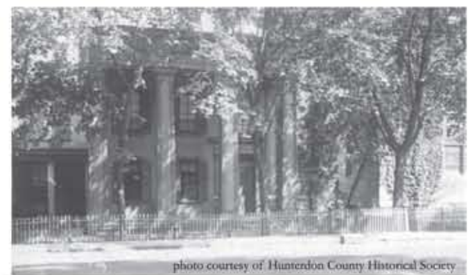
14 Doric House/Mahlon Fisher residence 1846 Fisher built his Greek Revival style home utilizing many of his trademark architectural elements: decorative grilles for attic ventilation, oversized columns, Greek wreath motifs and specialized moldings.
